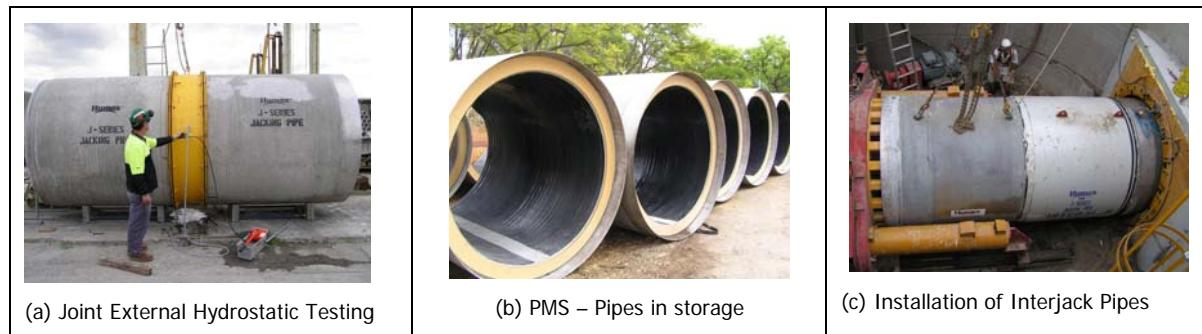
**Photograph 1 - Jacking Pipe Testing, Storage and Installation**
