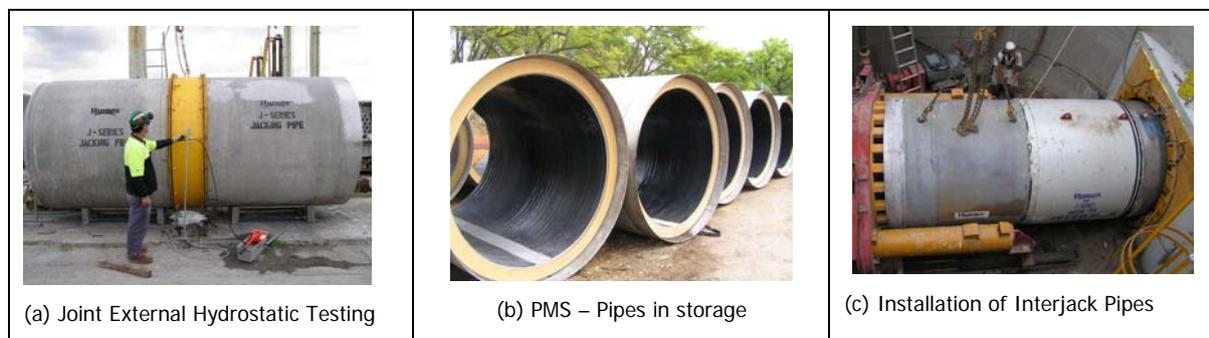
**Photograph 1 - Jacking Pipe Testing, Storage and Installation**
