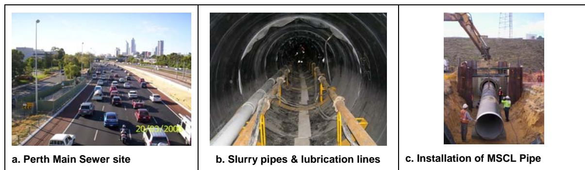
**Photograph 2 – Construction of Jacked Pipelines**
